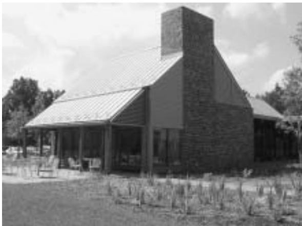
The New Henry Wallace Visitor’s Center that Gateway staff cleans. Located on FDR site in Hyde Park, NY
